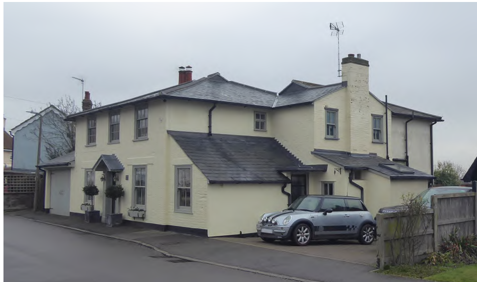
Figure 28 The Saltings, Manor Road
