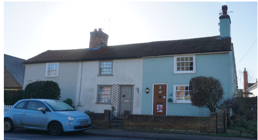
Figure 24 Numbers 1-3 Chapel Cottage, Colchester Road
