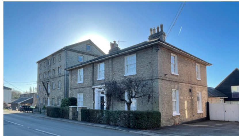
Figure 27 Mill House and Phoenix Mill
