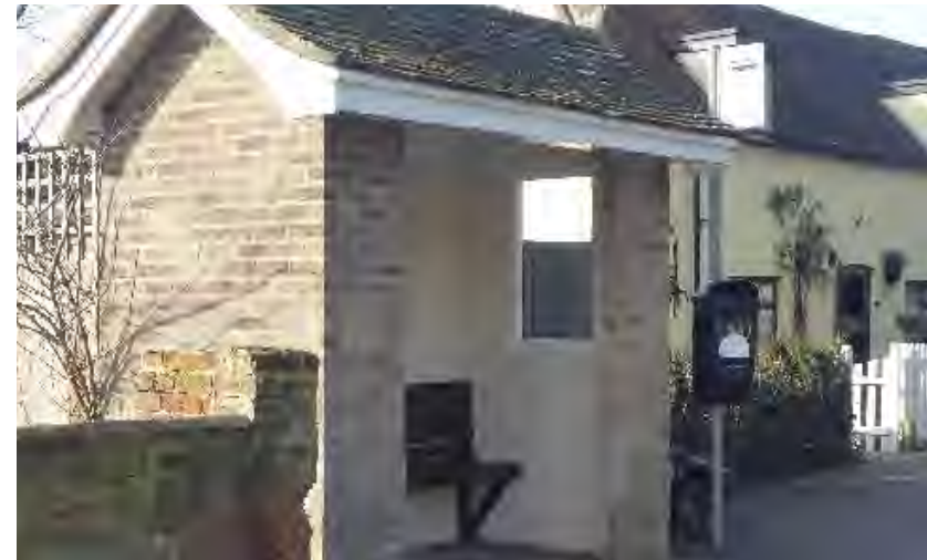
Figure 52 The bus shelter on Rectory Road
