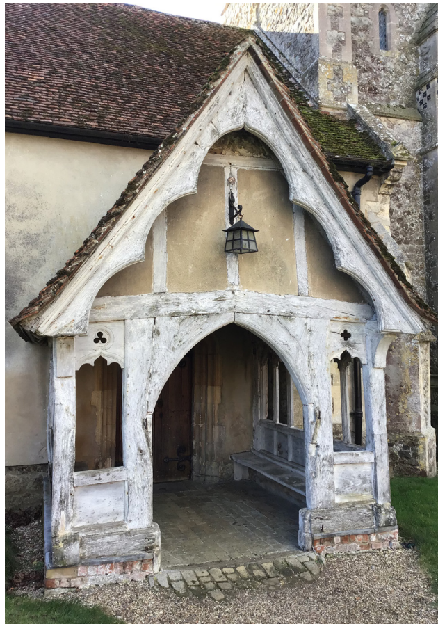
Figure 21 Fourteenth century timber north porch at St Edmund's Church
