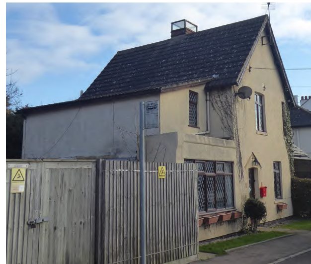
Figure 58 Ivy Cottage on Rectory Road
