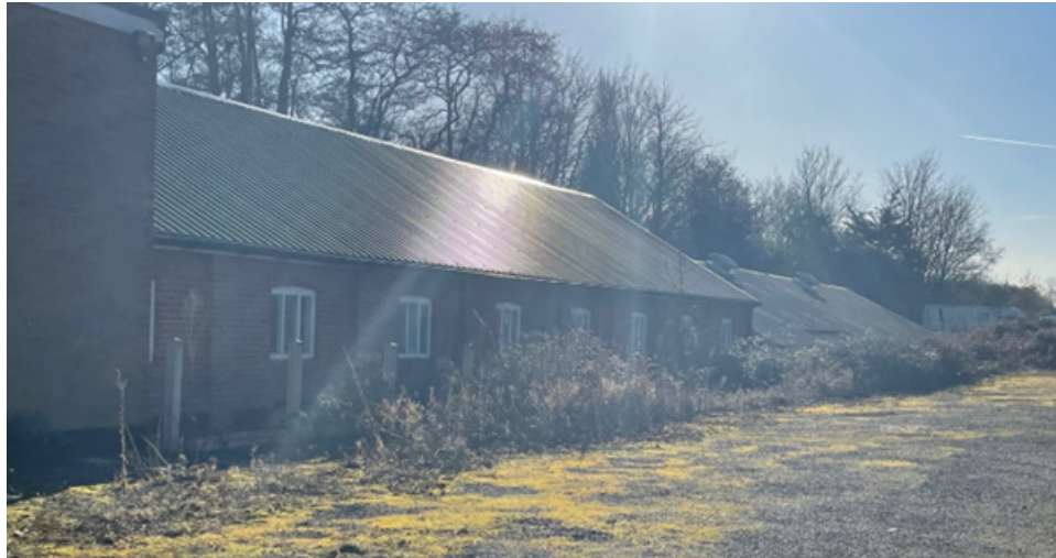
Figure 31 Ardleigh Studios (former goods sheds)
