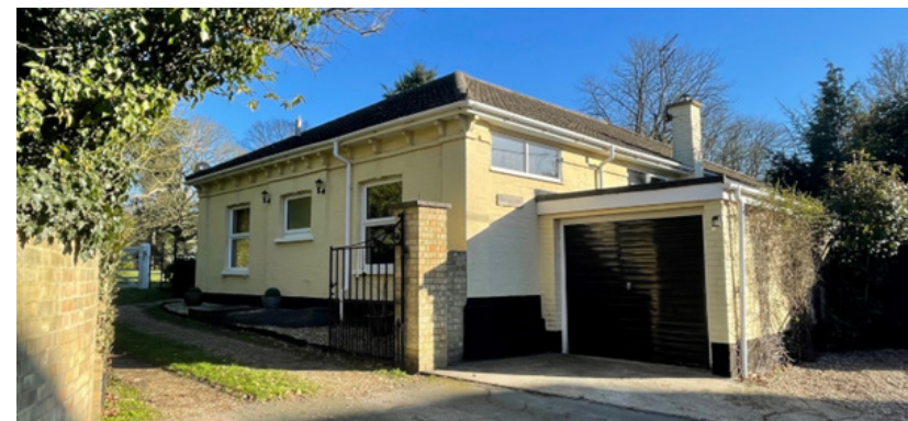
Figure 34 New Hall Lodge
