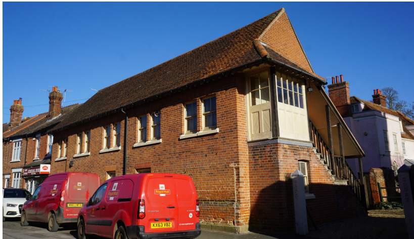
Figure 21 Church Hall (west of The Vicarage)
