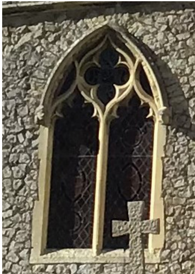
Figure 24 Stone and flint wall with limestone dressing at St Edmund's Church
