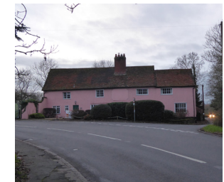
Figure 15 Grade II Listed Crown House
