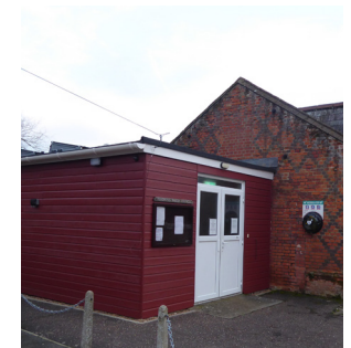
Figure 41 Side extension at the Village Hall clad with fibre cement boards
