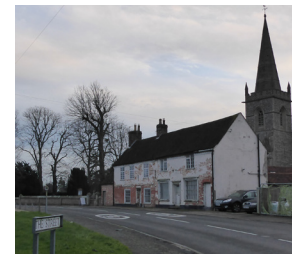
Figure 16 Grade II Listed 1 The Street (Church Cottage)
